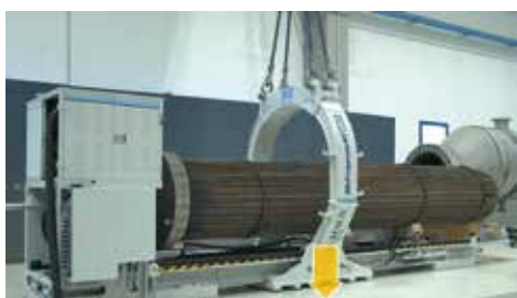
Release from shell and depositing on ground using a crane 6
