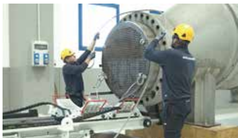
Anchoring to the shell 1
